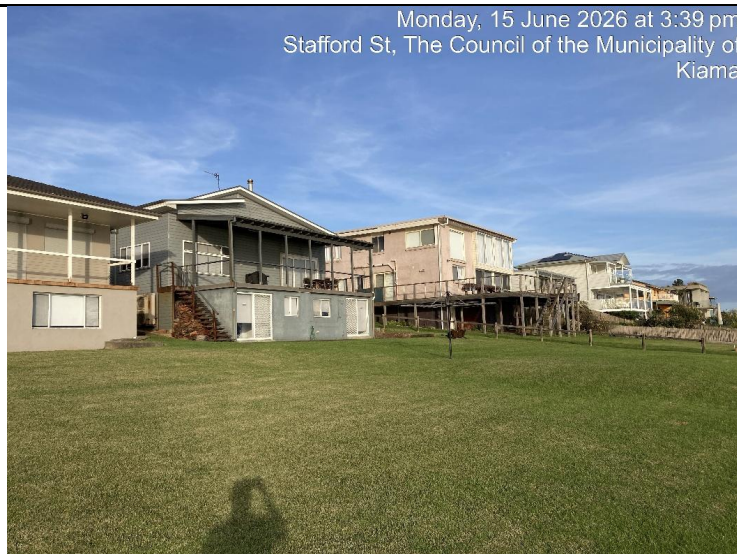
Figure 2: Photo looking East over subject site towards eastern adjoining site.
