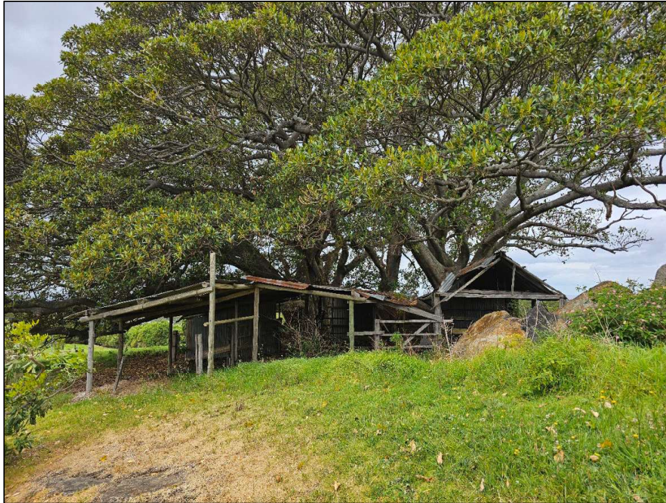
Photo 9 – The remains of former shed structures beneath the Moreton Bay Fig. The structures use old and modern building materials and would require significant works and replacement of original fabric to restore them.
