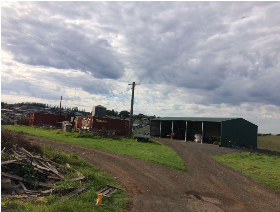
Figure 16: Site Photo of onsite machinery sheds
