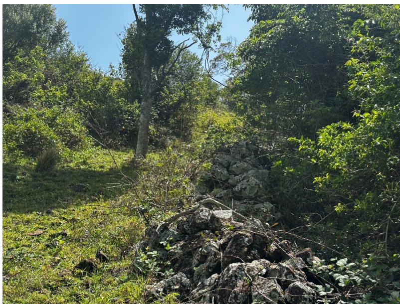
Figure 54 View of dry stone wall [14] within the central portion of the study area, facing east
