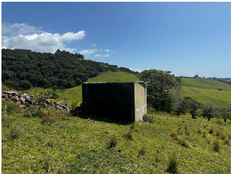
Figure 48 View of the concrete structure [24] near the western boundary dry stone wall [4], facing north-west
