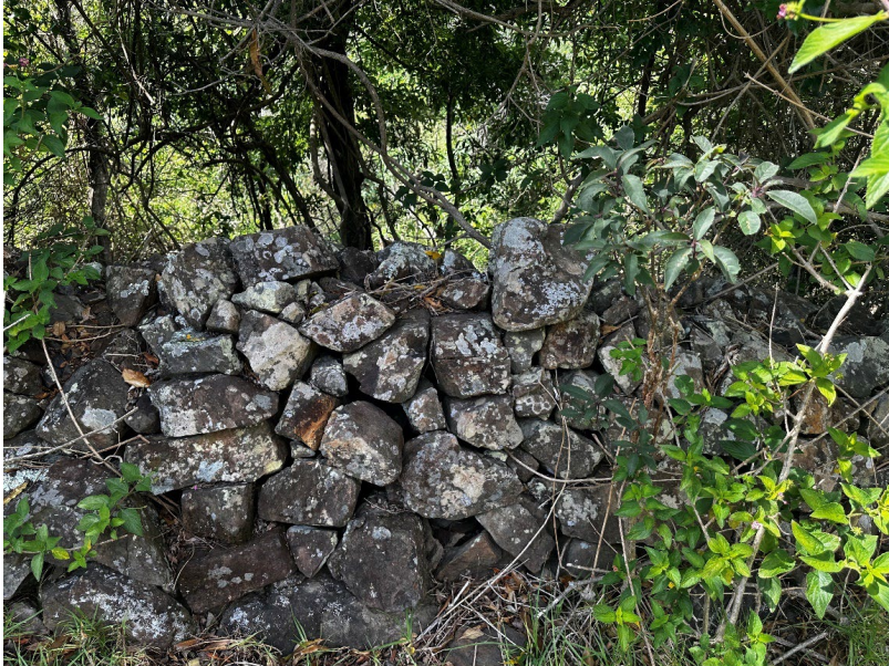
Figure 55 Detailed view of the existing condition of dry stone wall [14]
