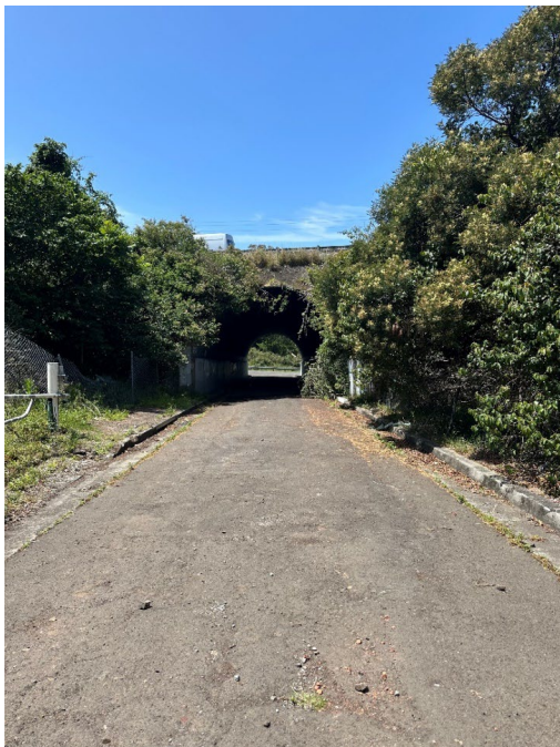
Figure 28 View of the arched underpass of the Princes Highway from the farm entry, facing east
