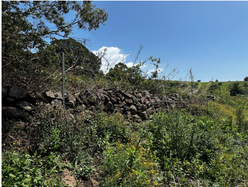
Figure 45 Existing condition of the western boundary dry stone wall [4], facing north
