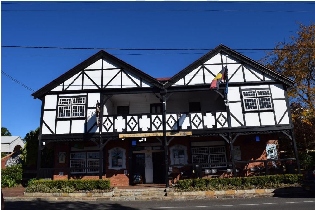
Figure 7: Jamberoo Hotel facing Allowrie Street, view looking south.
