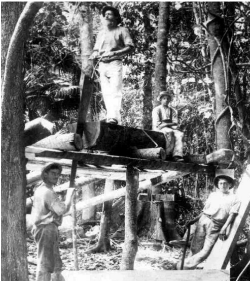
Plate 1: An early cedar sawpit constructed over a creek (source: A prelude to: The History of Jamberoo).
