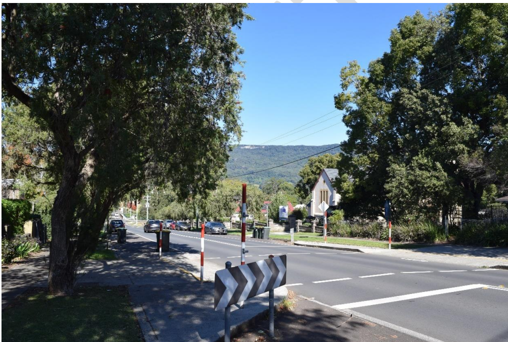
Figure 3: Jamberoo Anglican Church located along Churchill Street, view looking southwest.
