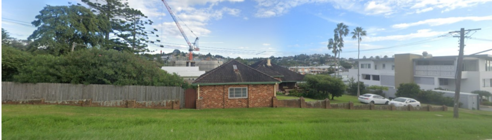
Figure 3 – Site Photograph – existing dwelling on No 21 Bourrool St looking west
