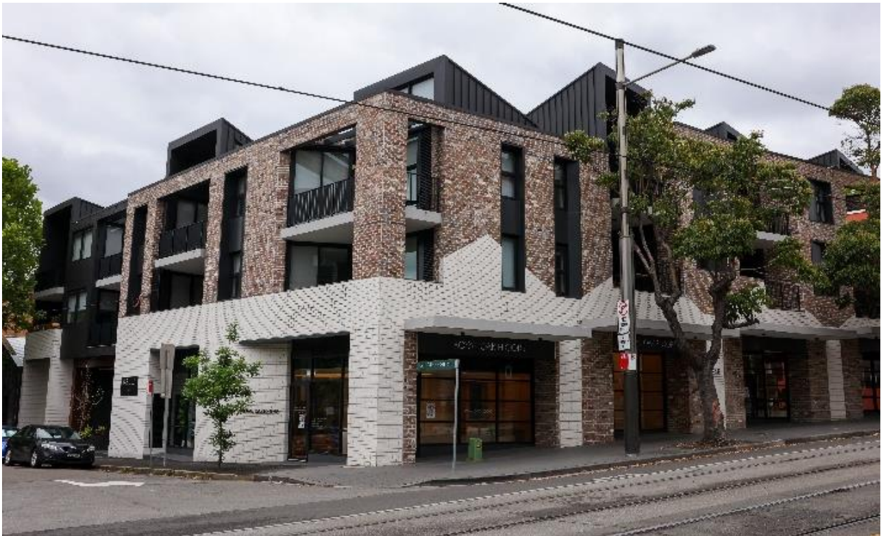
Figure 4: Shop top housing in Surry Hills
