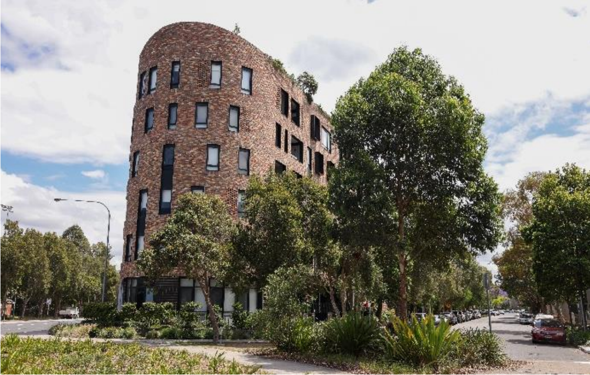
Figure 4: Residential flat building on Huntley Street, Alexandria
